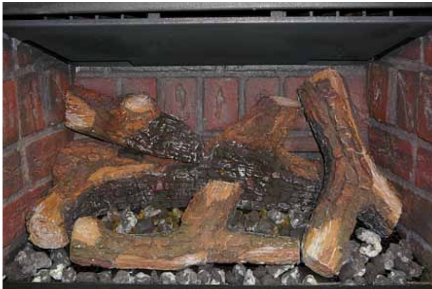
Figure 50. Log Set and Ember Installation.
