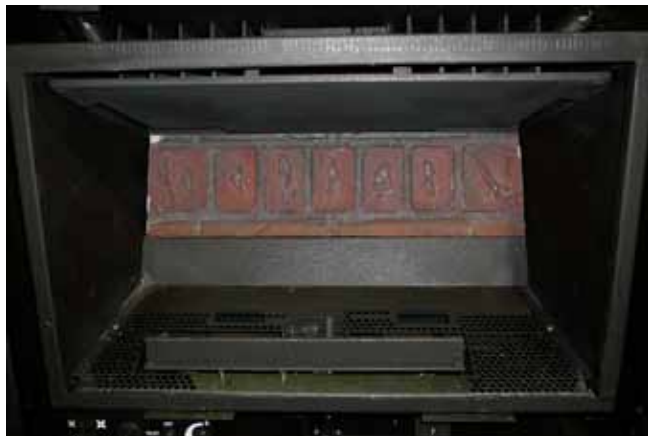
Figure 42: Back Brick Panel in Place.
