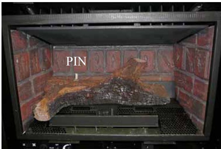
Figure 45. First Stage Log Set Installation.
